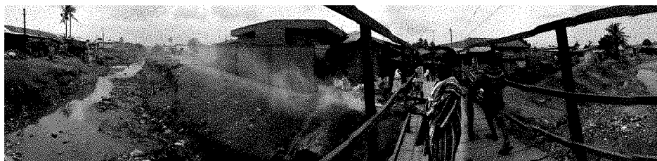
Photo 3: An Open Drainage Channel in a Low-income Neighbourhood Photograph by Michael Donovan
